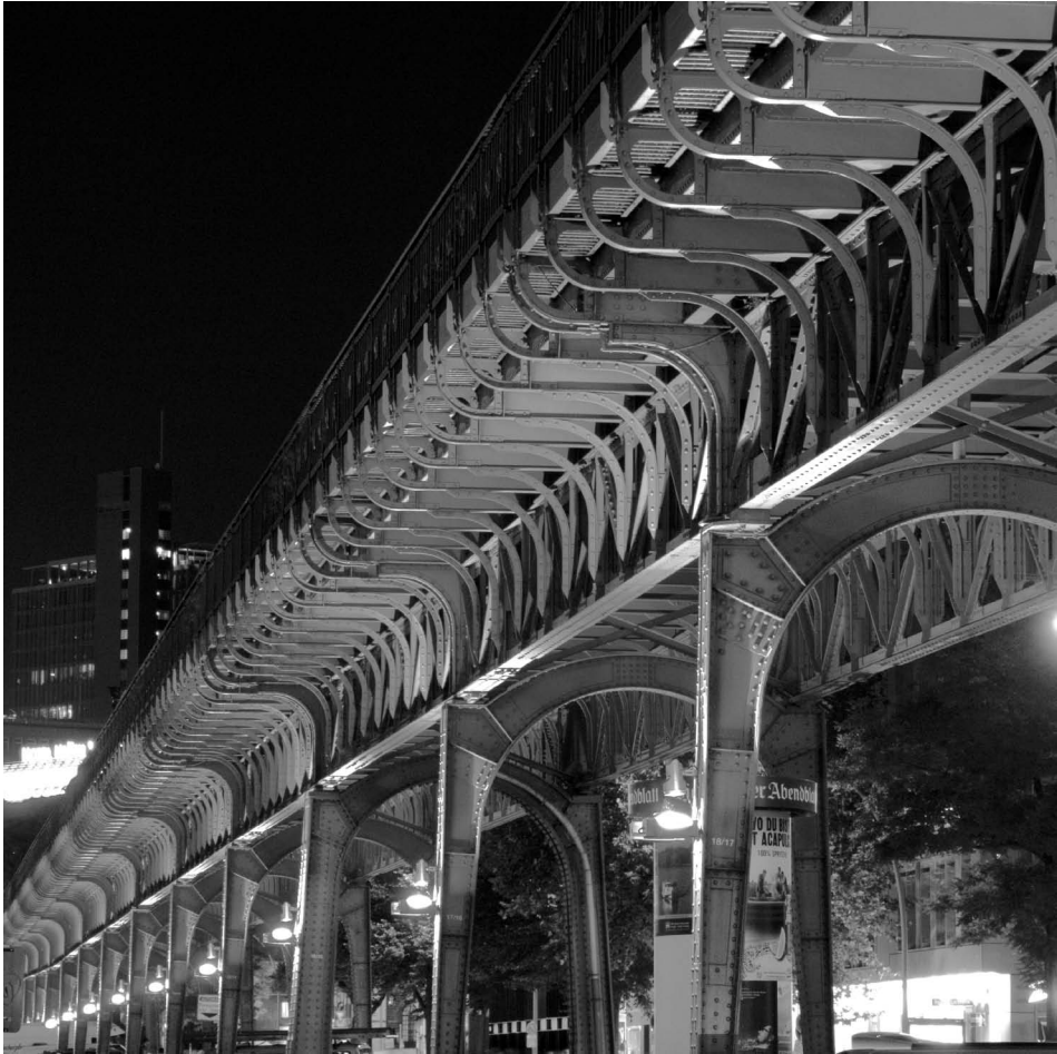
Abb. 2 U-Bahn-Brücke am Baumwall in Hamburg
